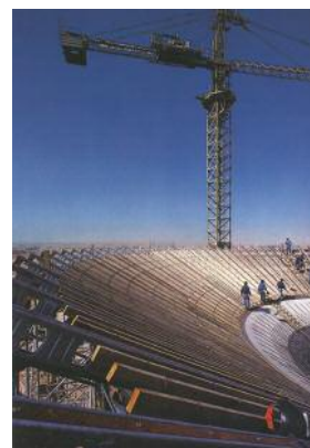
Enormous water towers under construction.
